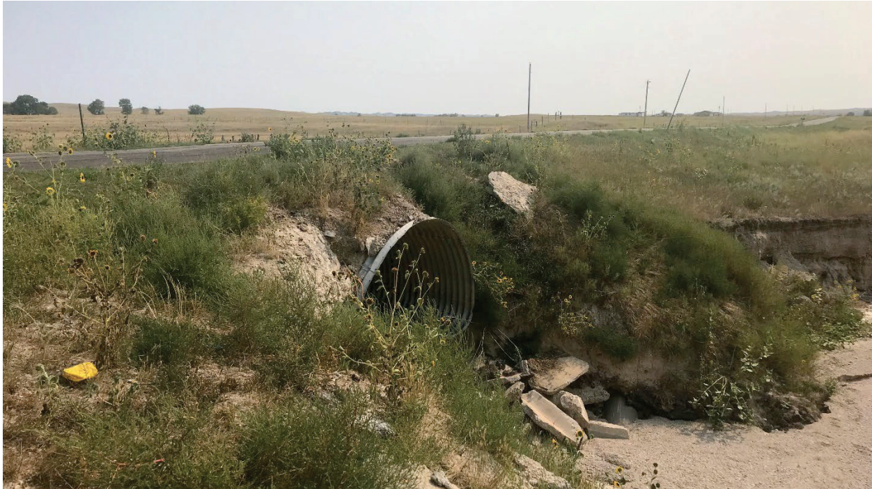
Figure 22: Existing Culvert on BIA 33
