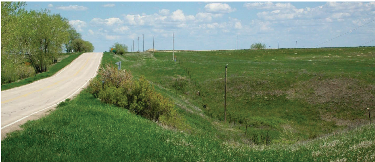
Figure 23: Typical Steep Embankments along Culverts
