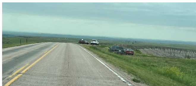
Existing Red Shirt Overlook is Dangerous Adjacent to BIA 41
