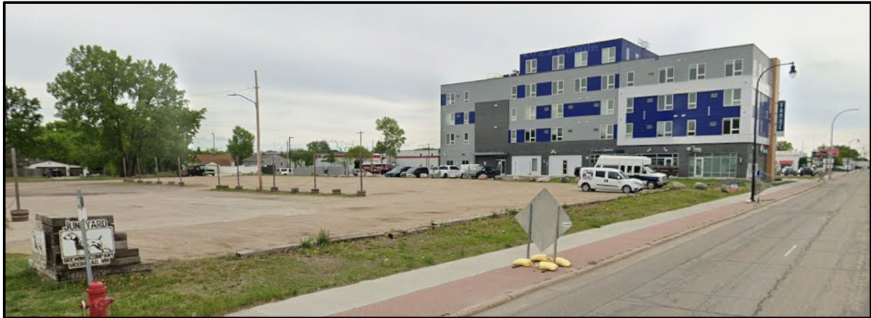
Figure 26: 1st Avenue at 15 Street N looking northeast
